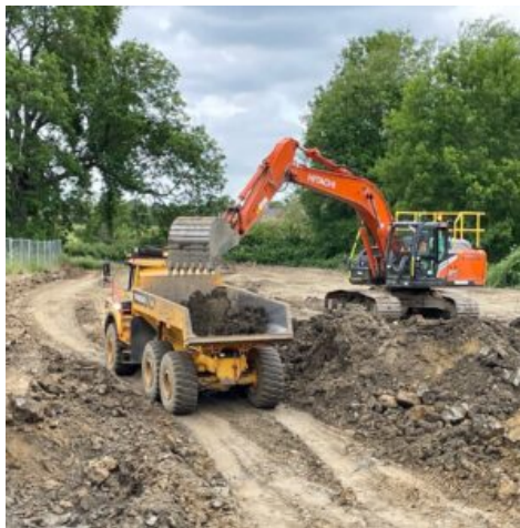
Construction work on a Davidsons Homes site in Fleckney, Leicestershire
